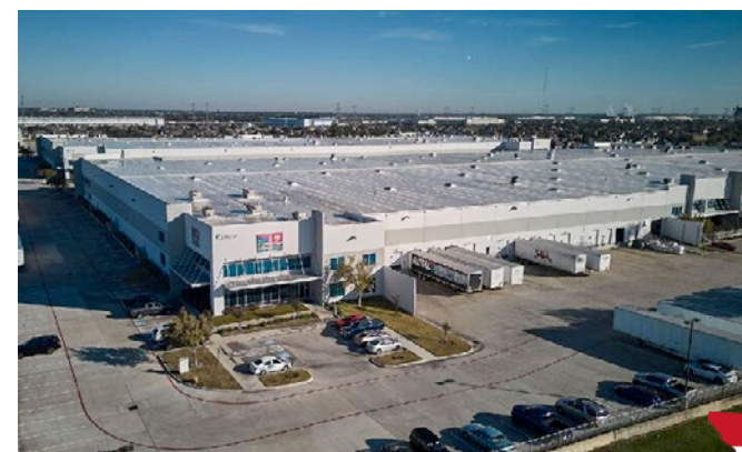
At the Rittal Application Center in Houston, customers can see the future of panel building and switchgear manufacturing for themselves and try out applications.
